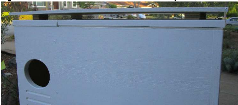
Figure 2: Installed Sun Shield
